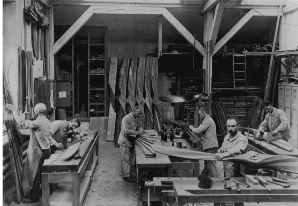
Propeller production in the former K+W in Thun (today RUAG), under license from Wild.
